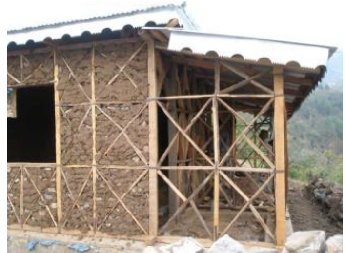
Mud and stone infill ; Dhaji-dewari technology
