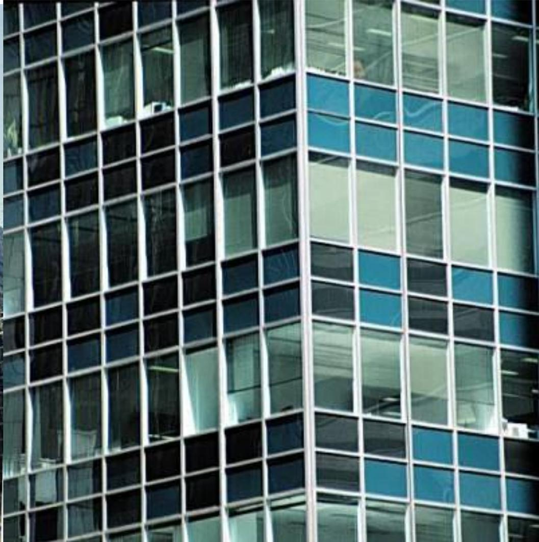
**DGU: Insulating glass** consists of two or more sheets of glass separated by a hermetically sealed air space.
