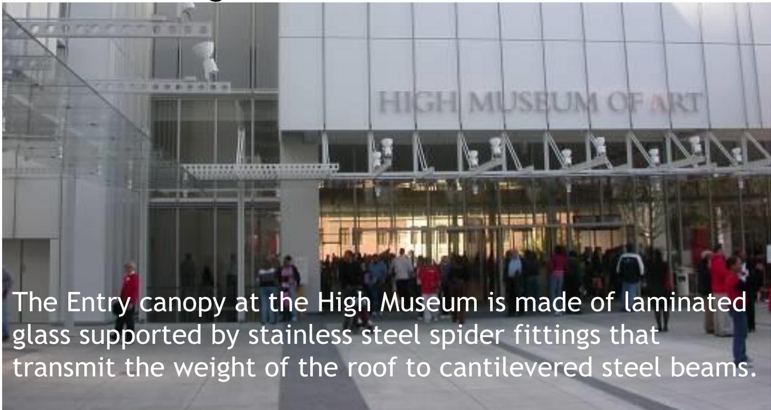
The Entry canopy at the High Museum is made of laminated glass supported by stainless steel spider fittings that transmit the weight of the roof to cantilevered steel beams.
