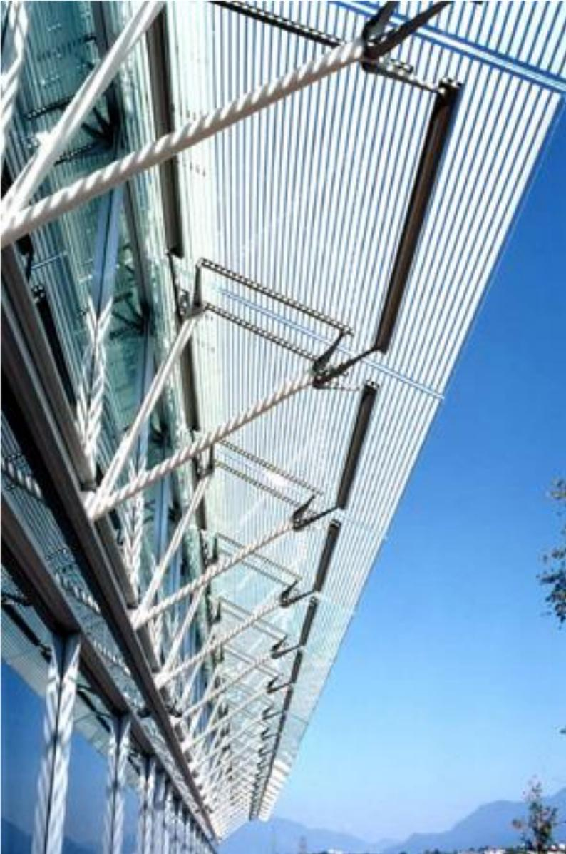
Glass that has an imprint on the surface with silk screened patterns of ceramic based paint. Paint is fired in a glass furnace to transform into a hard ceramic permanent coating.
