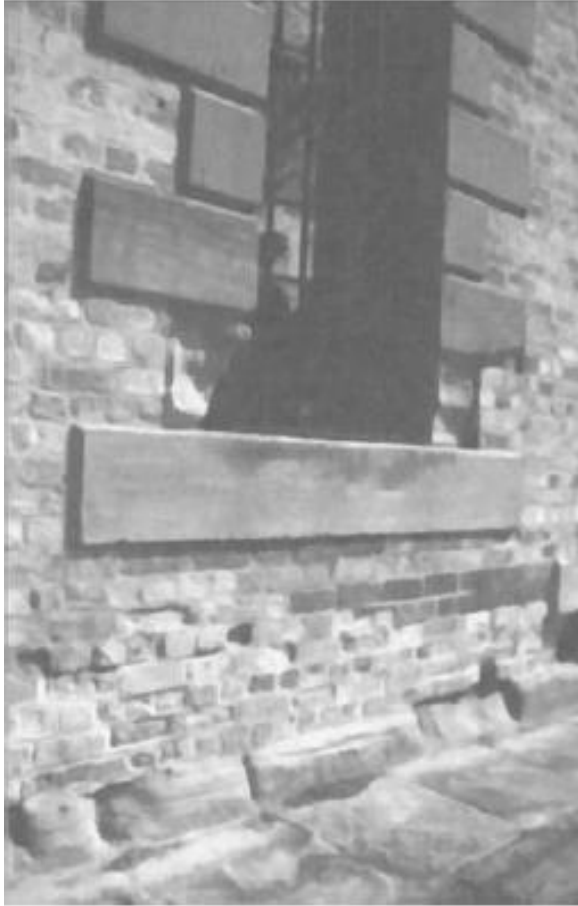
Rising damp in brick and stone masonry. Note how the worst decay is at the base of the window opening. This is where most evaporation takes place and hence most decay due to salt attack.
