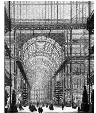
Figure 5.23 Interior of London’s Crystal Palace, the Construction of Which Was Inspired by the Leaf Structure of the Amazon Water Lily
